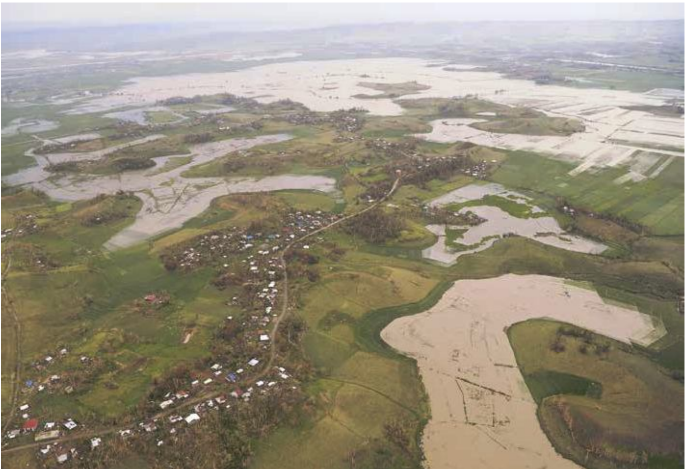
Damaged Homes and rice and corn fields by typhoon Mangkhut in Alcala, Philippines |
