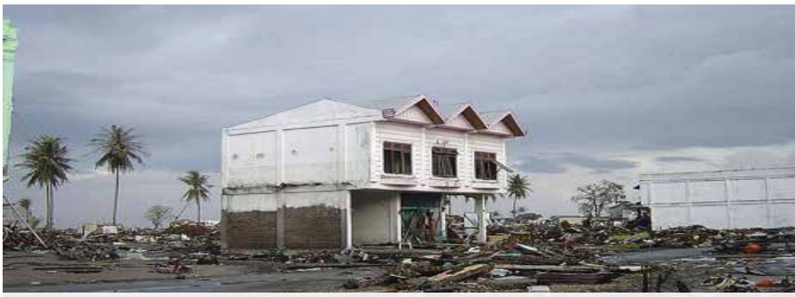
Damage in Banda Aceh During 2004 tsunami | Source: US Military
