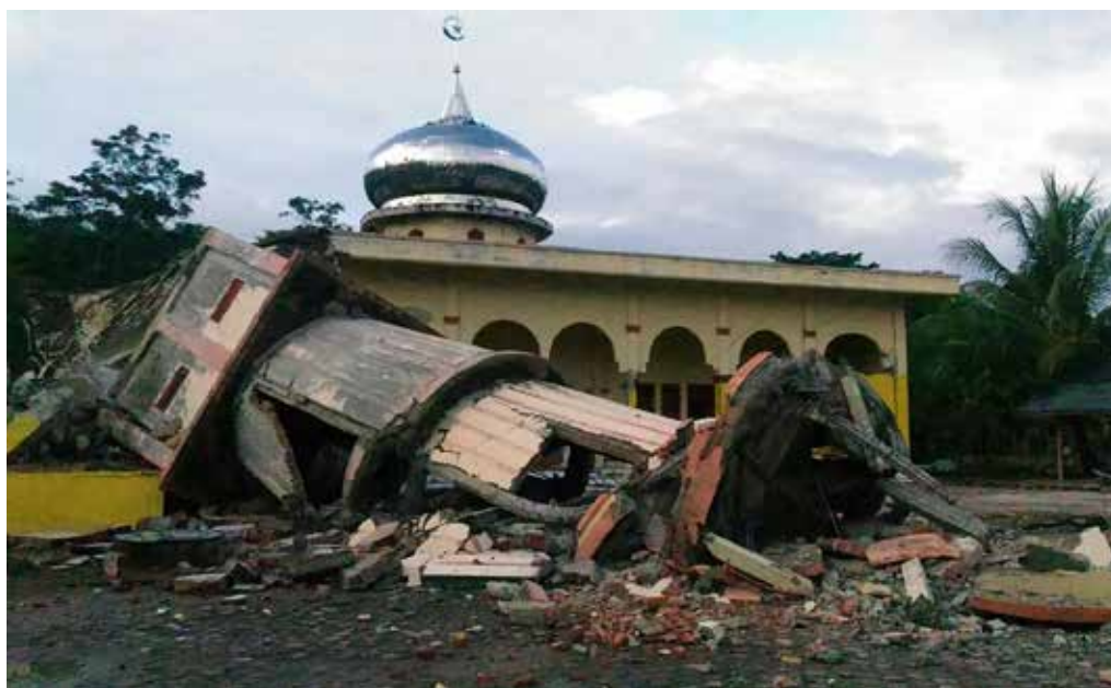
Damaged building during Dec 7, 2016 EQ in Aceh, Indonesia | Source: The Independent
