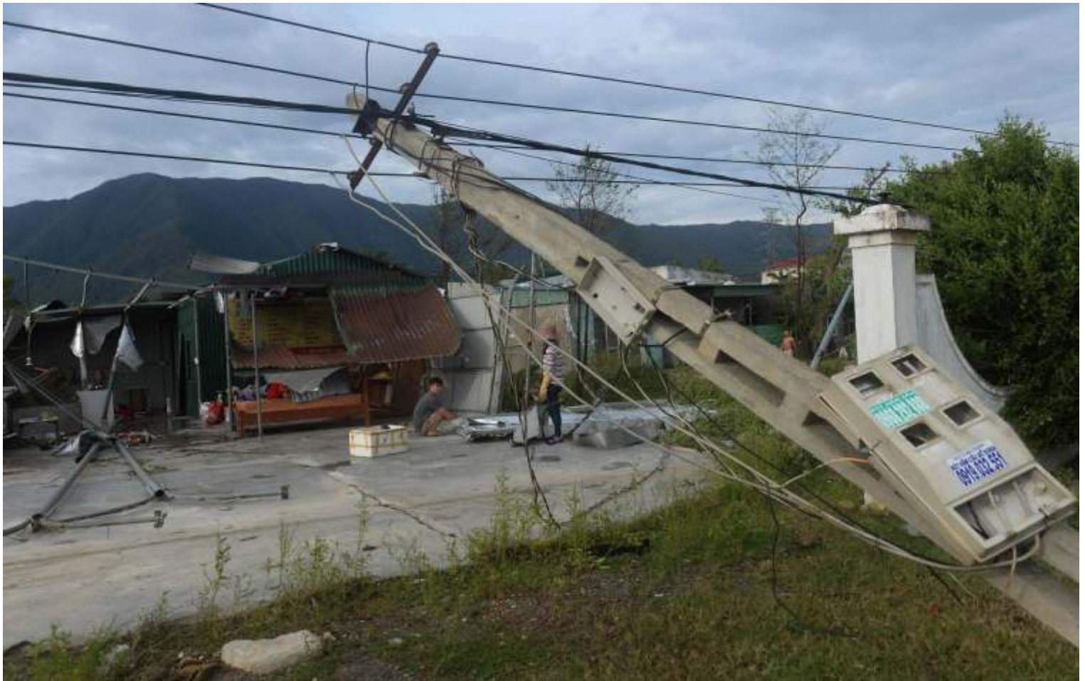
Damaged home next to a broken pole and cables in Ky Anh town during typhoon Doksuri 2017 Source: saigoneer.com
